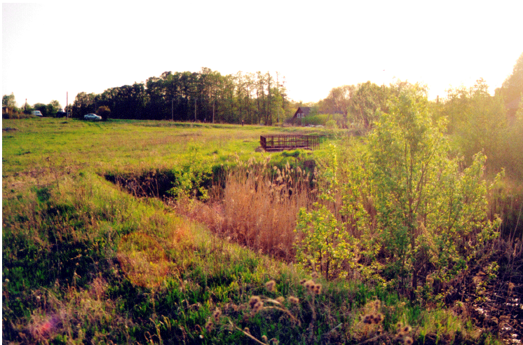
The old bioponds at Vohnja will be reconstructed and isolated from the ground with biomembrans
